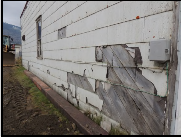
Asbestos shingle siding with shiplap underneath
